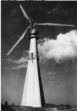
Figure 4: three-bladed F.L. Smidth machine, built in 1942. Source: Windpower
